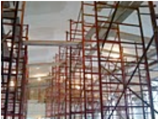
Patching and Plaster Nearly Complete
