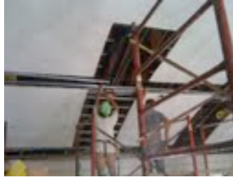
Furring Begins to Close Ceiling Holes
